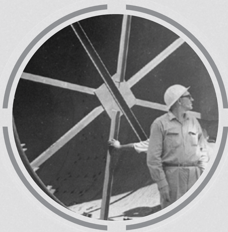
CONSTRUCTION OF THE FIRST PLANT IN SANTA HELENA, BRAZIL
